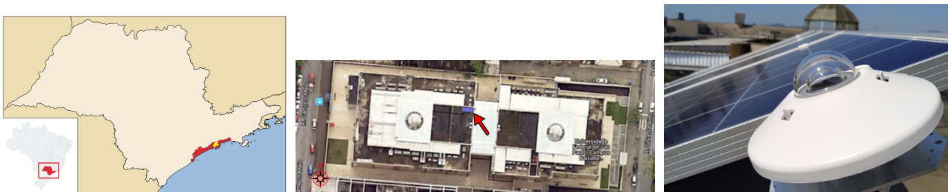
Fig. 1. Location of the installed PV system, in Santos, coastal city in the Brazilian Southeastern region. The central image shows the Unifesp's rooftop where the PV and data acquisition systems (right) are operating.
